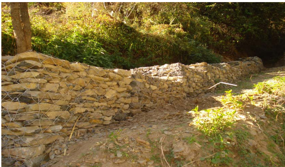
Crate work executed under NREGS in GP Mangla, Block Mehla
